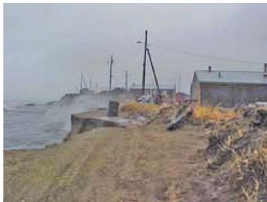
Figure 1. Shishmaref, AK. Erosion from winter storm surges required the village to be relocated. Source: Shishmaref Erosion & Relocation Coalition
