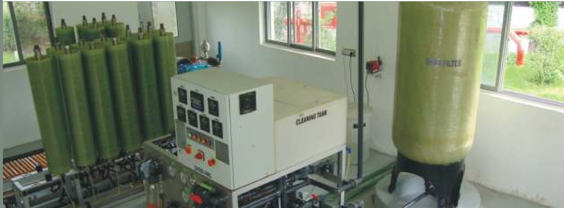
Reverse Osmosis plant
