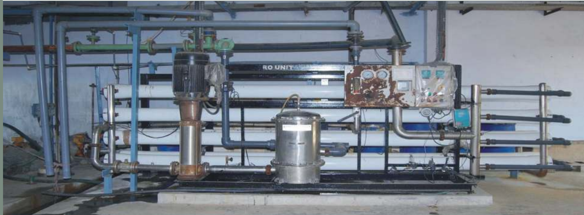
Reverse Osmosis plant
