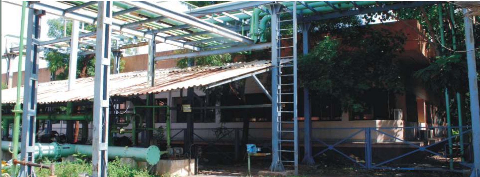
Overhead water circulation system
