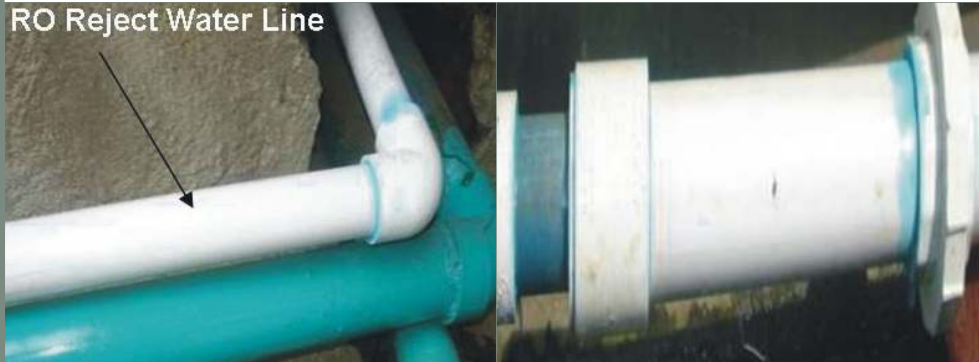
RO reject water line
