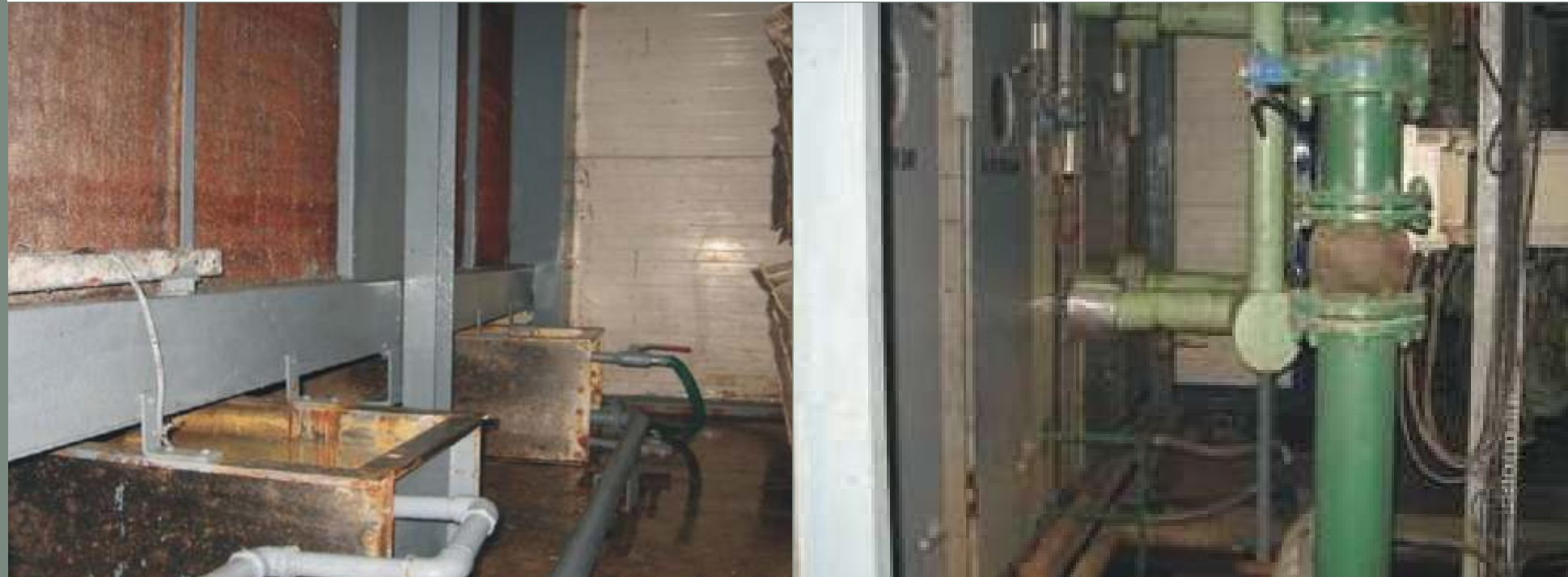
Air Handling Units
