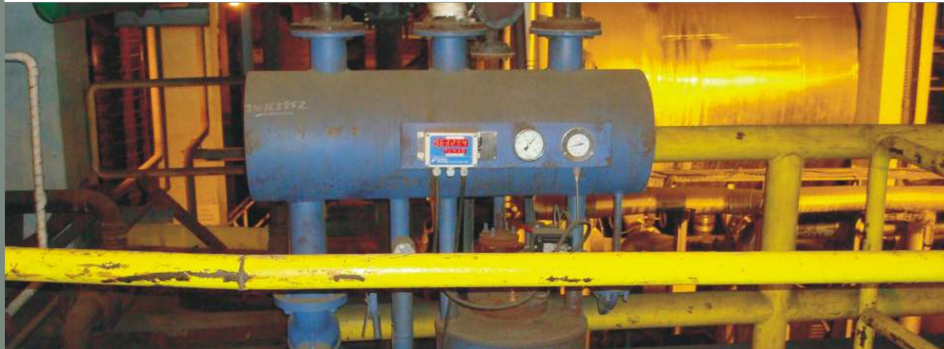
Condensate recovery pump
