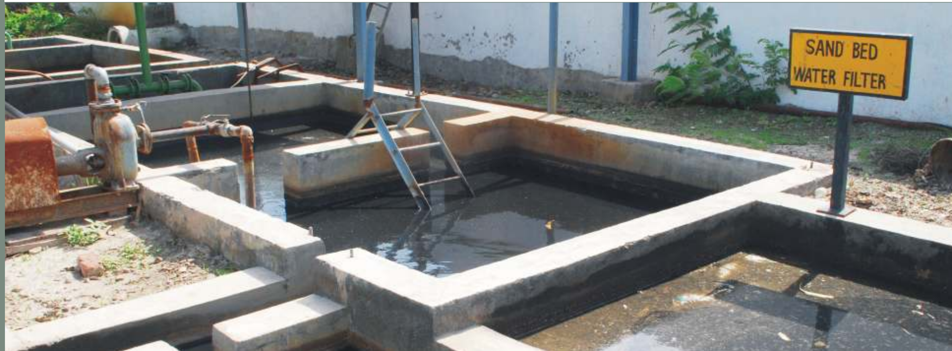
Wastewater tanks used for cullet washing
