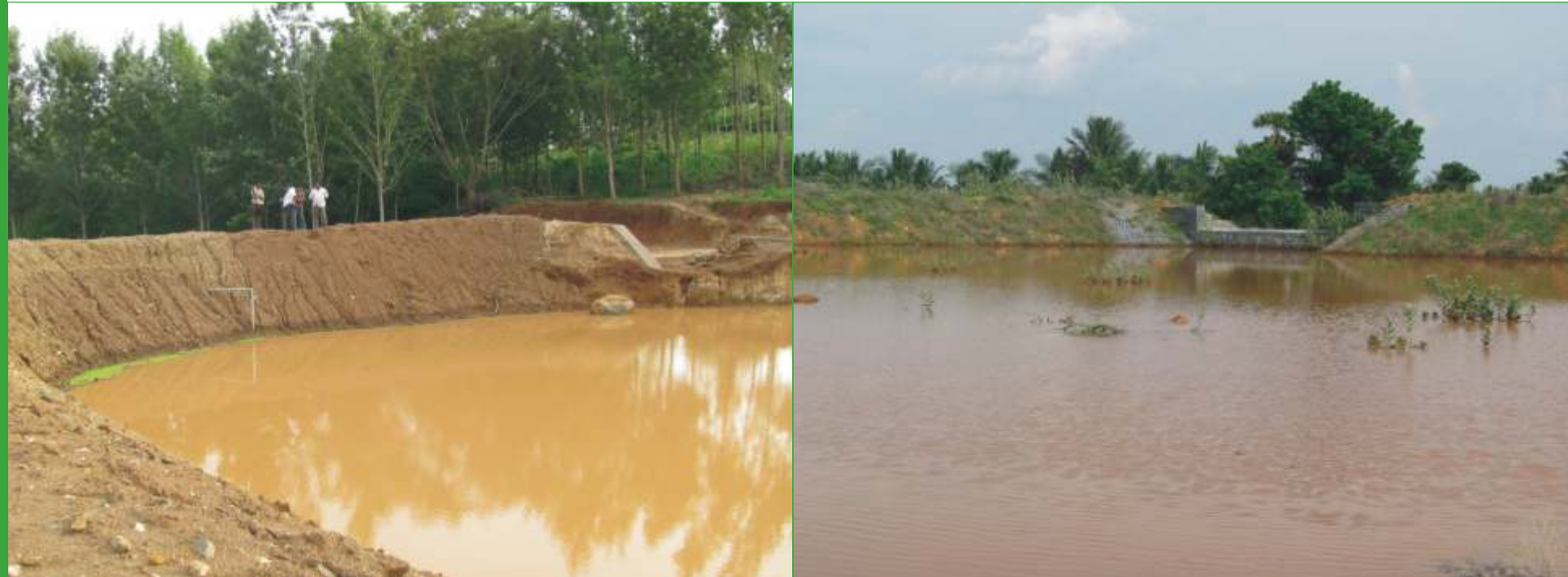
Rain Water Harvesting structures
