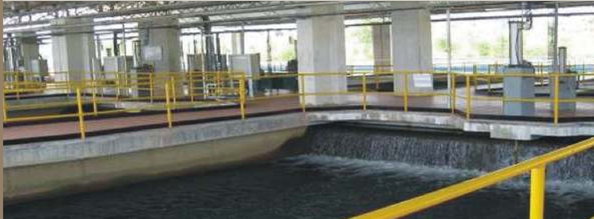
Drinking water treatment plant
