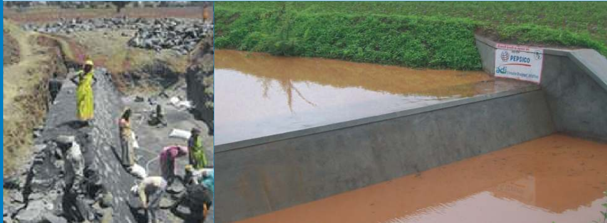
Check dam during construction
