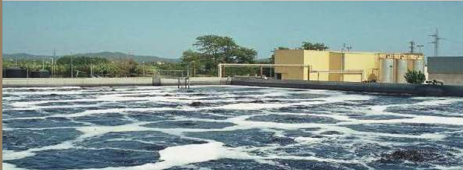
Common effluent treatment plant
