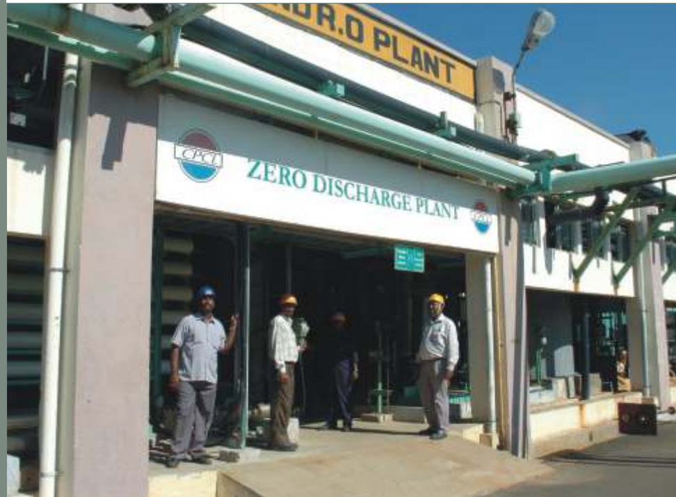
Zero discharge plant
