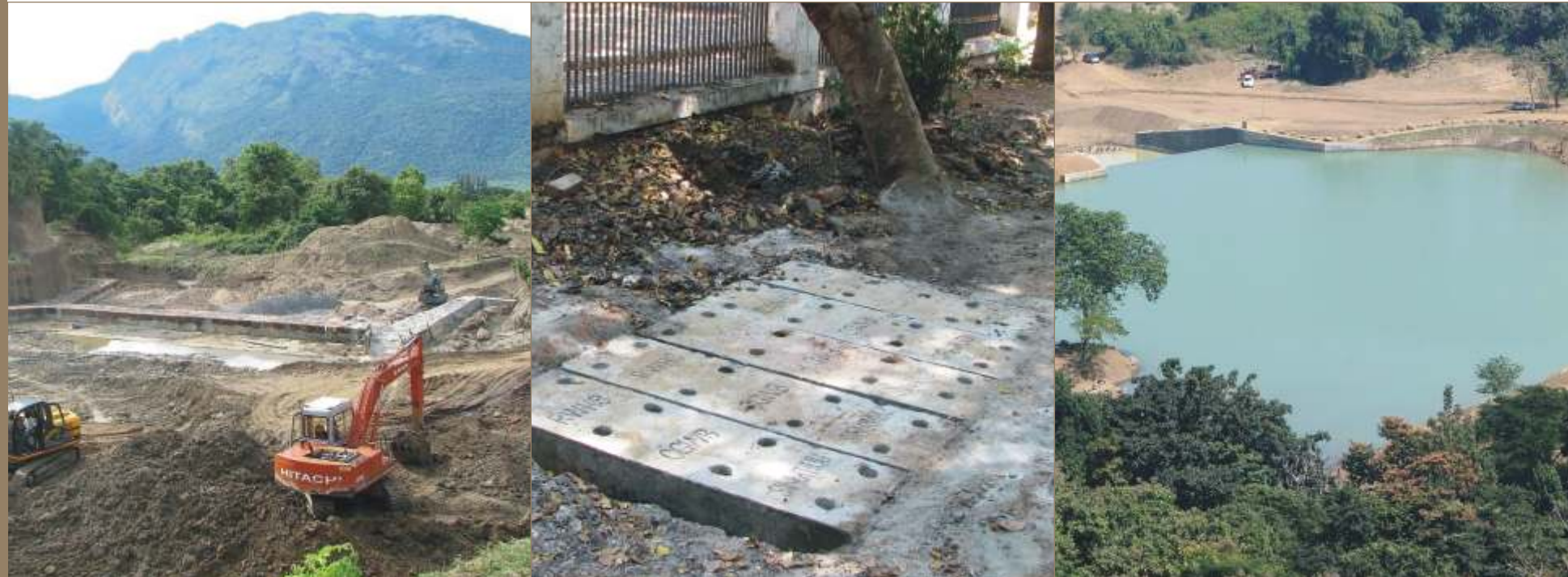
Work in progress - Nandangarai check dam
