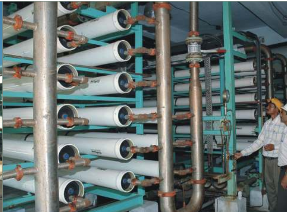
Reverse Osmosis and Ultra Filtration plant
