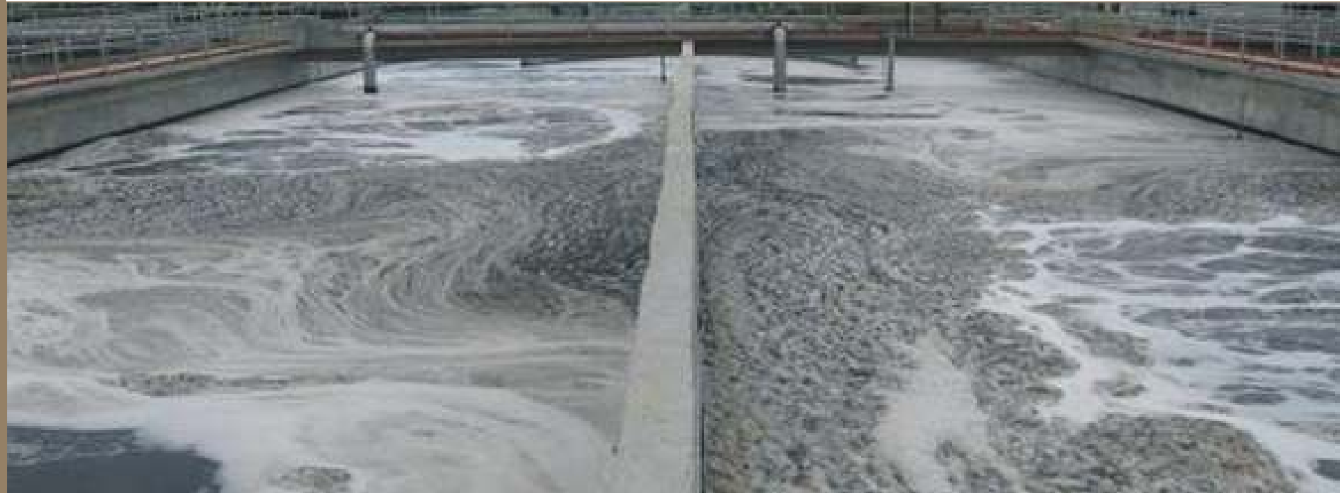
Common effluent treatment plant
