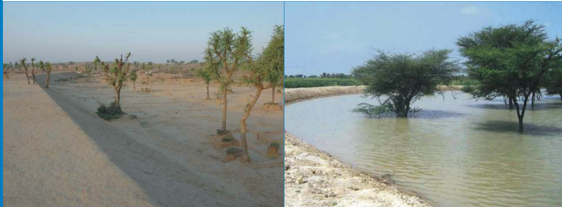
Constructed water harvesting structure before rainfall
