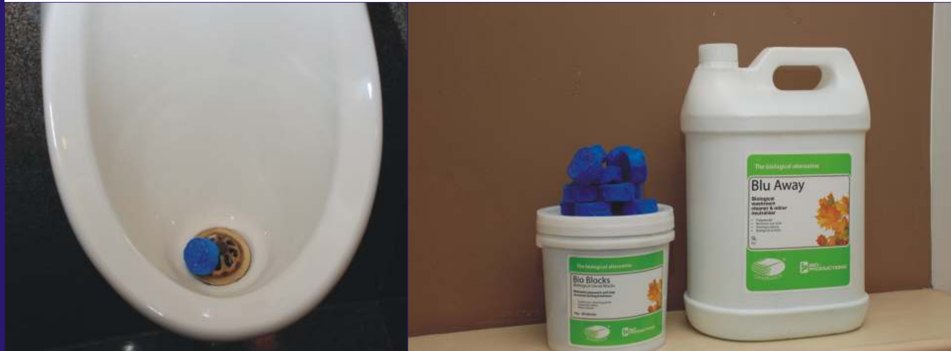
Waterless urinals with bio blocks
