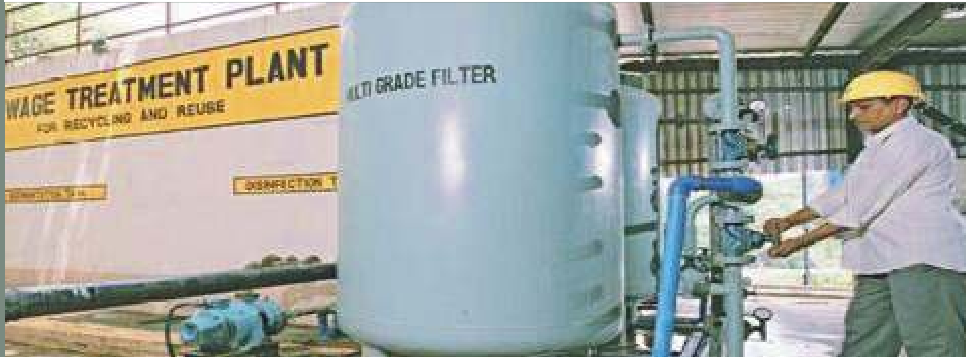
Sewage Treatment Plant
