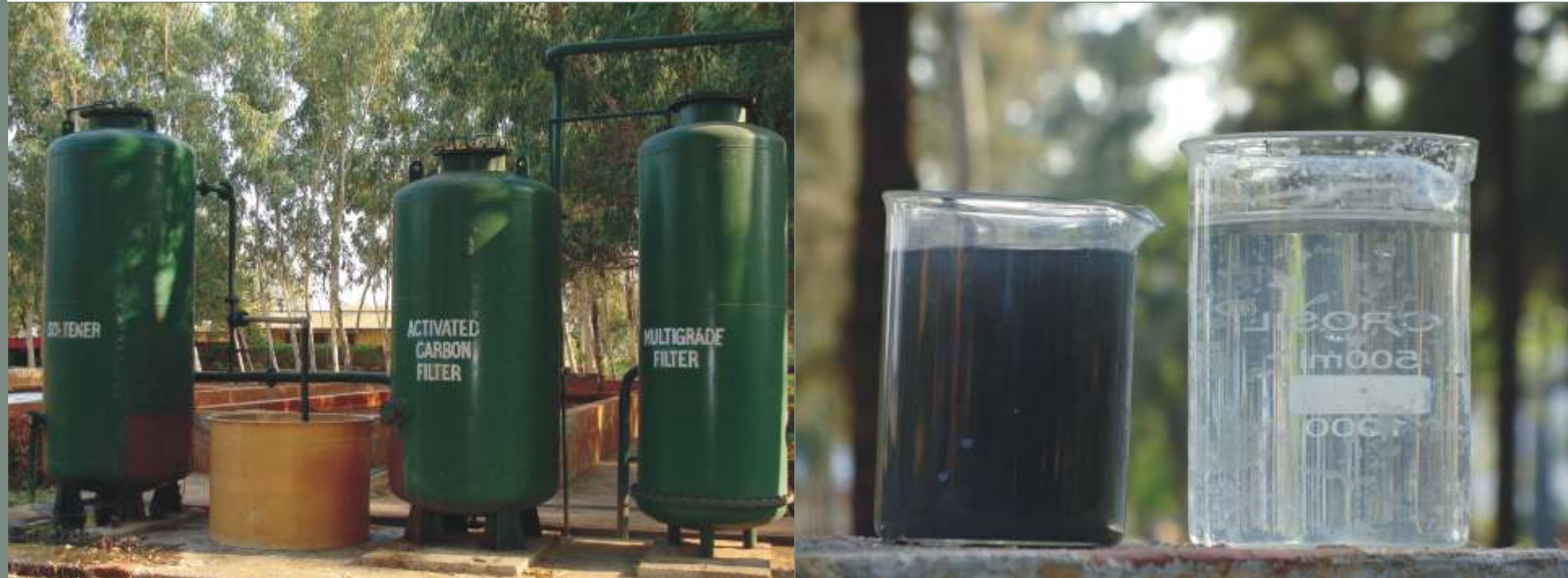
Wastewater treatment plant
