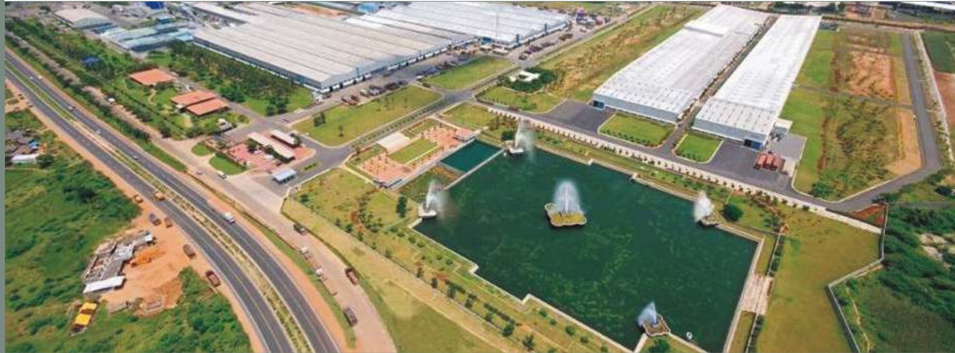
Water reservoir for storing rain water
