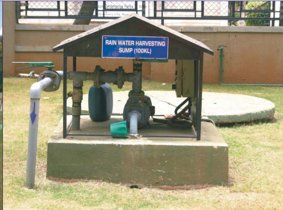
Rain Water Harvesting sump
