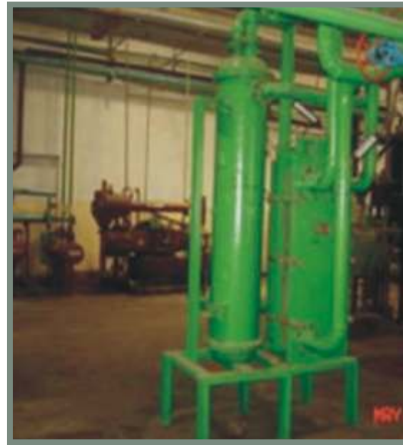
Plate heat exchanger
