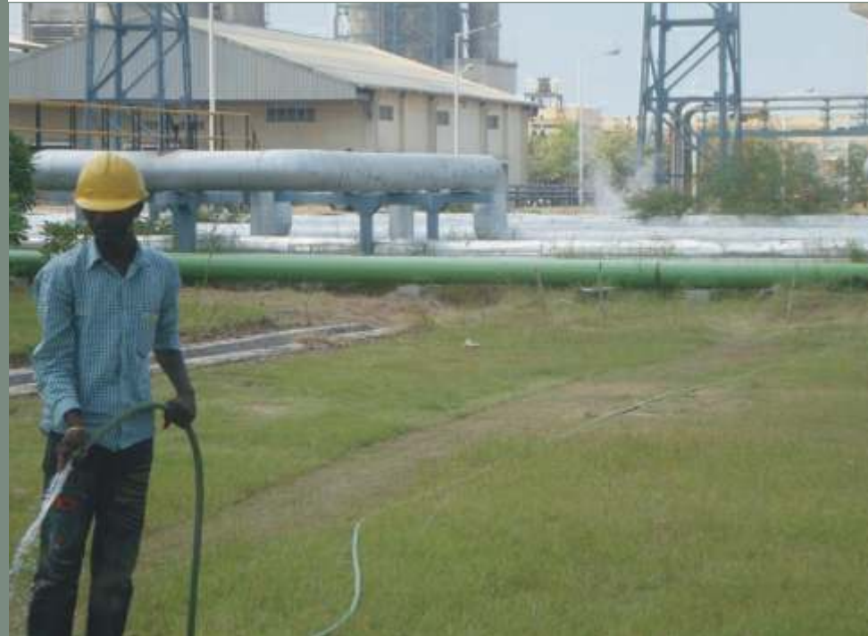
Cooling tower blow down water used for gardening
