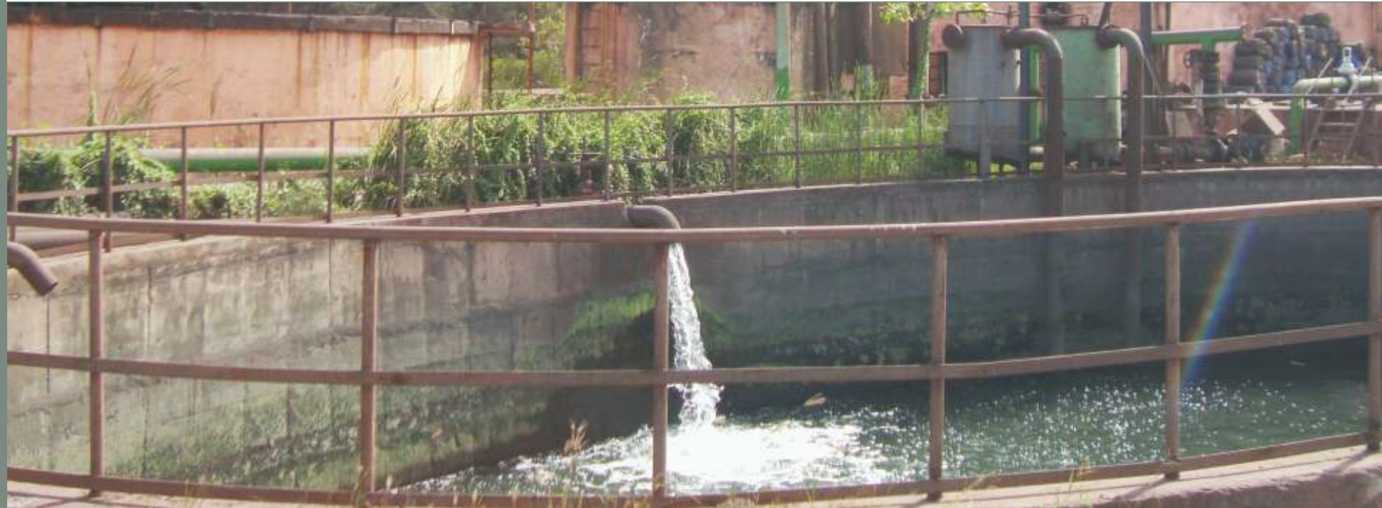
Pond for collecting cooling tower water
