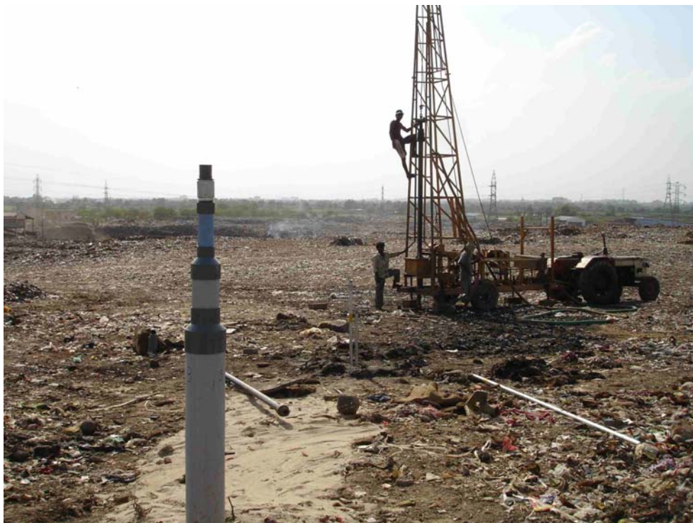
Figure 3-4. Pump Test Extraction Well and Drill Rig
