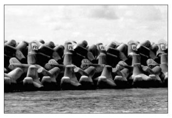
Figure 7: Tetrapod Technology is extensively in use in Maldives. The picture shows a Tetrapod wall protecting a coastal slope. (Courtesy: R. K. Bhandari)
