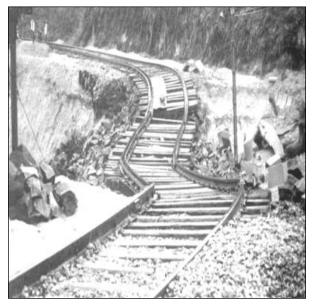
Figure 14: The more than 100 year old Watawala Earthslide in Sri Lanka was completely controlled through use of innovative subsurface drainage technology. Despite this, no other SAARC country has used this technology to control similar landslides. (Courtesy: R. K. Bhandari)
