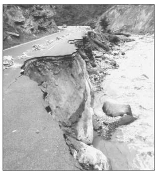
Figure 3: Breach of a stretch of highway that occurred on 26 May 2009 at Km 143.23. (Courtesy S. S. Porwal)
