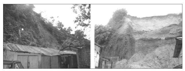
Figure 4: Showing the landslide happened due to hill cutting for construction purpose
