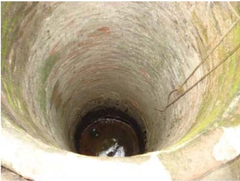
Lowering of water level of surface wells due to excessive sand mining in the area.
