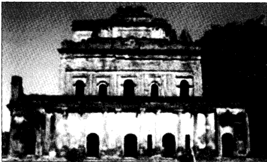
Figure 2. Monuments constructed with snail lime during Ahom dynasty in Assam: (top) Rang Ghar, (middle) Tolatal Ghar, and (bottom) Kareng Ghar (Photo credit: Kharkhuwa; www.google.com ).
