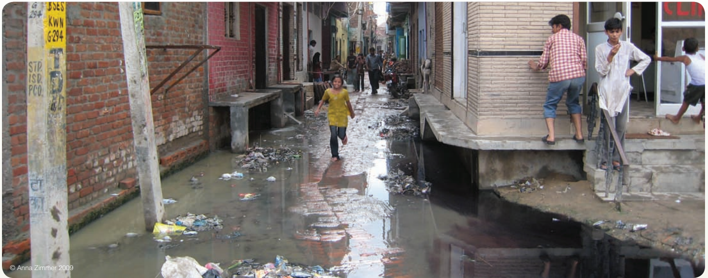
Wastewater drains in an unauthorized colony
