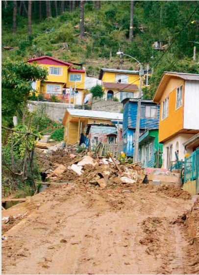
Figure 4: Landslide in Argüita de la Perdiz, Chile. Source: P. Aldunce
