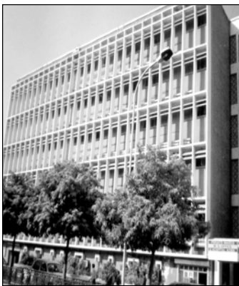
Fig. 1: A typical multi-storeyed Building
