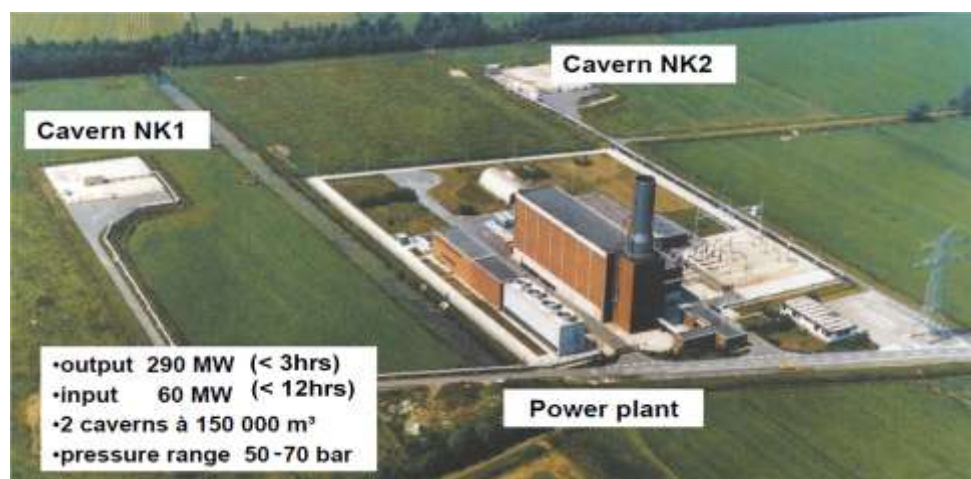
Figure A.23: Aerial view of Huntorf
