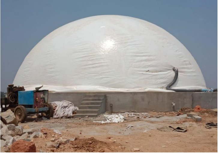
Methane Collection chamber
