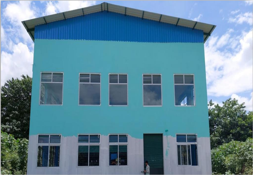
Decentralized Dry Waste Processing Plant
