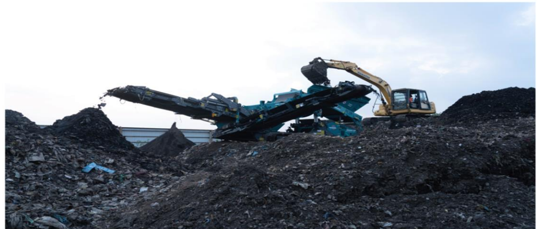
Work in Progress-HDMC CC, Dharwad Dt. – 50000 Tons remediated so far.
