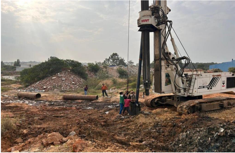
Installation of Methane Collection Pipe
