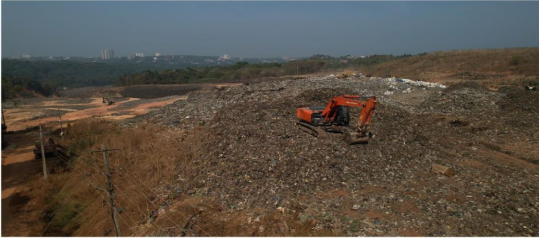
Work in Progress –Mangalore CC, Dakshina Kannada Dt. - 105441 Tons remediated
