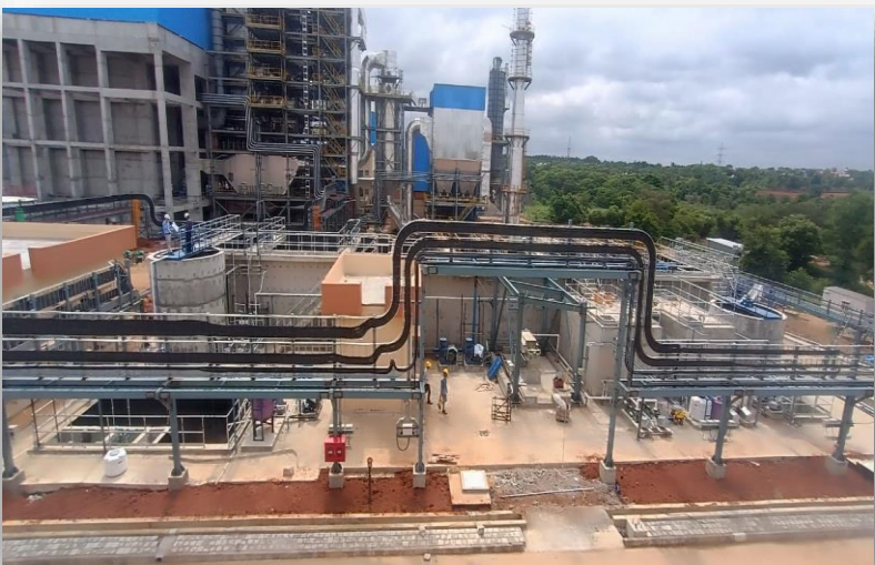
Constructed by KPCL to generate 11.5 MW of Power from 600 MTPD of RDF Waste
