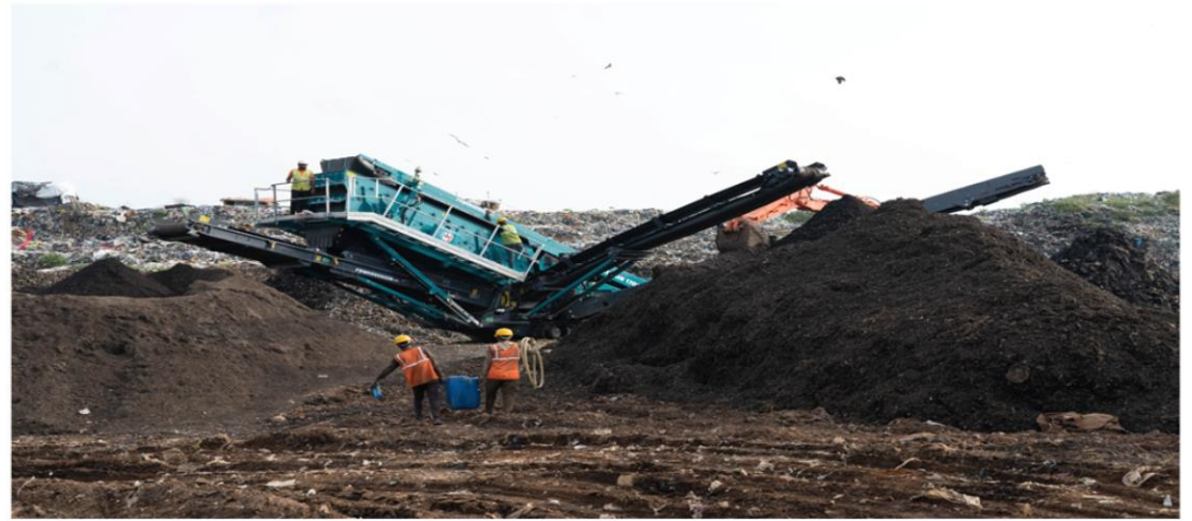
Work in Progress- Mysore CC, Mysuru Dt. - 160000 Tons remediated so far
