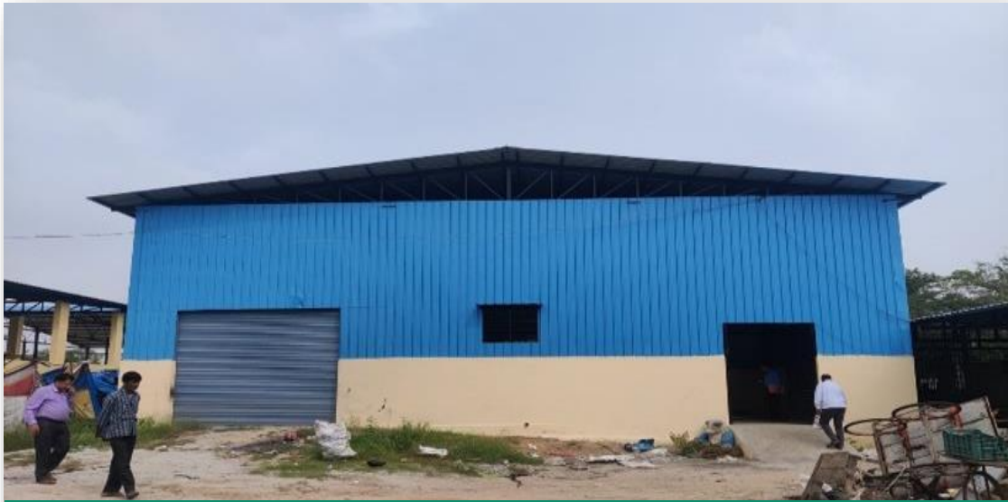
MRF Shed in T. Narasipura, Mysuru Dt.
