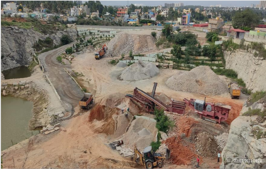
C & D Waste Processing Plant of capacity 750 MTPD established at Kannur
