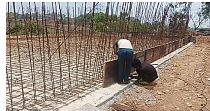
Foundation Work, HD Kote, Mysore Dt
