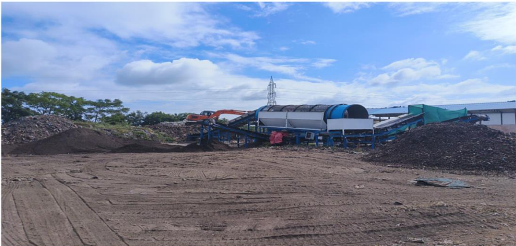
Work in Progress –Basavana Bagewadi TMC, Vijayapura Dt.- 22000 Tons remediated
