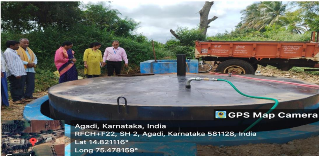
Biogas Plant of 60 cum capacity, Agadi GP
