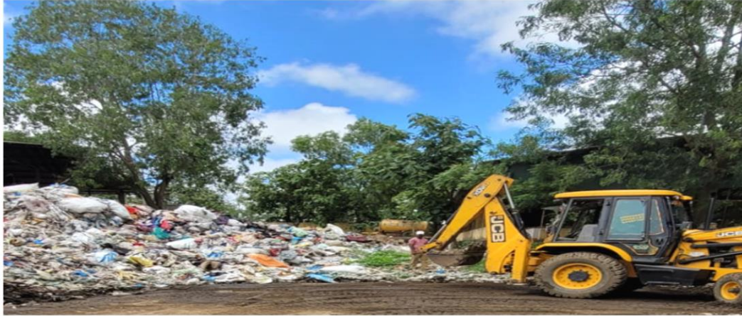
Before – Alnavara TP - 11,000 Tons of legacy waste
