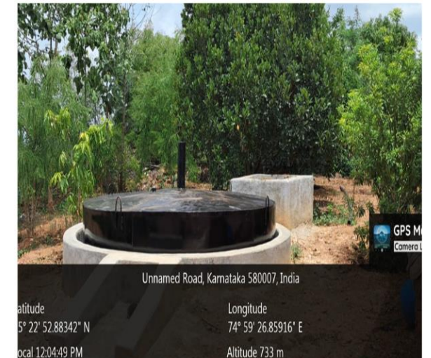
Biogas Plant of 45 cum capacity, Muthalli GP
