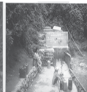
Potable Water Supply
