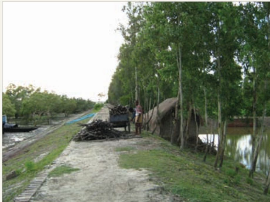
Embankments with gentle slope, wide tops, and mangrove vegetation in front withstood the onslaught of cyclone Aila
