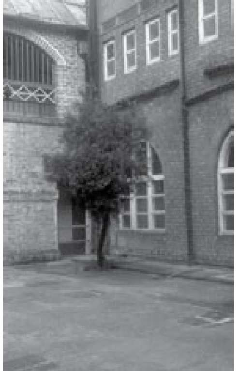
Underground storage tank
